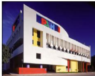
Regional Homeless Center 340 North Madison Avenue Los Angeles, CA 90004
